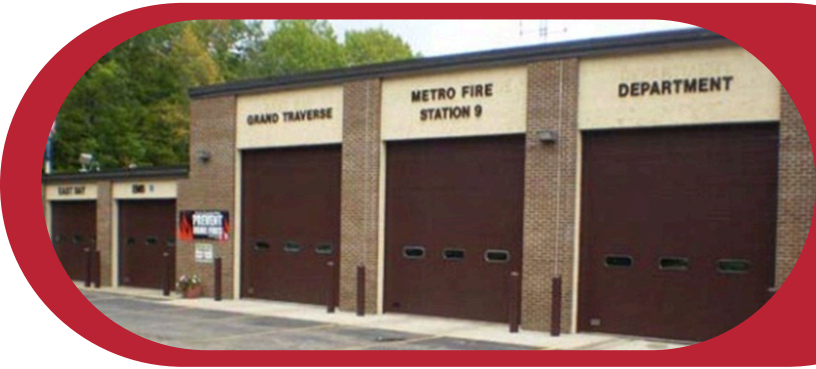
Station 9 | 110 High Lake Road (231) 947-0125
